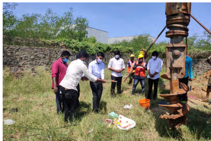
Stone laying ceremony of ARHC Projects in Sriperumbudur, Tamil Nadu
